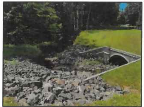
North Street Culvert Project – upstream side
