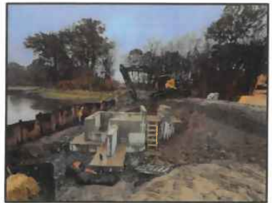
Nine Lot Dam Construction - Still Brook Park
