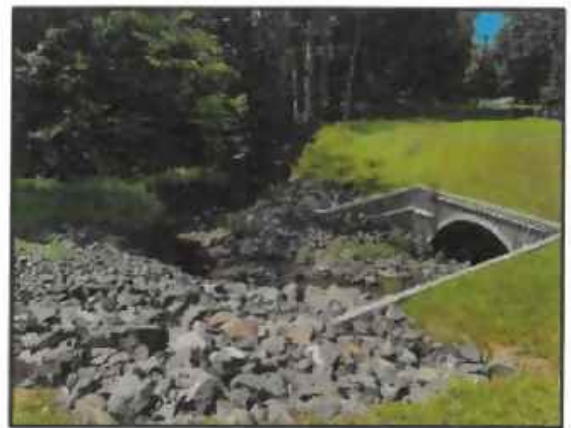
North Street Culvert Project – upstream side
