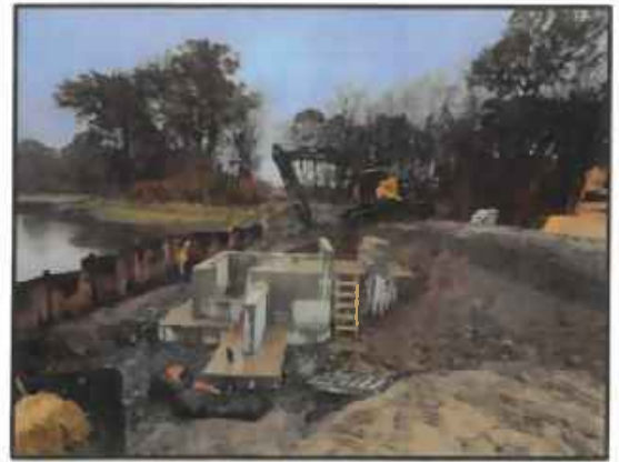
Nine Lot Dam Construction - Still Brook Park
