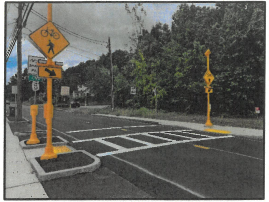
Rapid Flash Beacon - O'Brien's Corner - Springfield St
