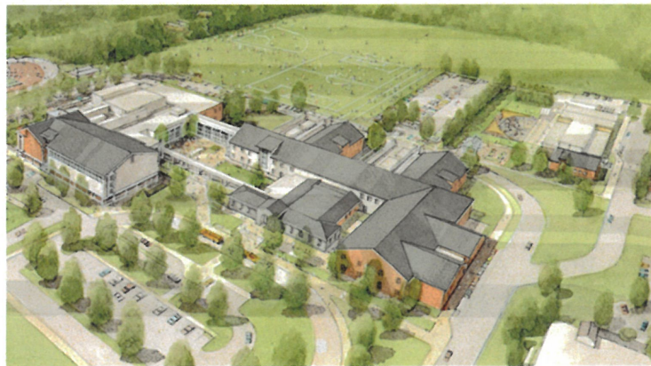
Agawam High School Project
