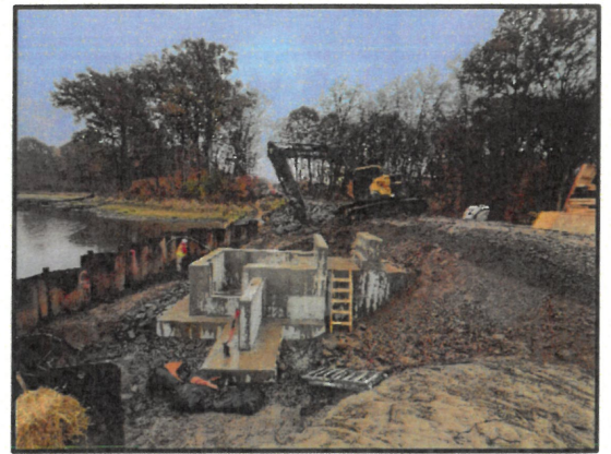
Nine Lot Dam Construction - Still Brook Park
