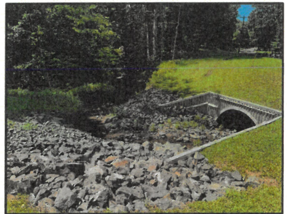
North Street Culvert Project – upstream side
